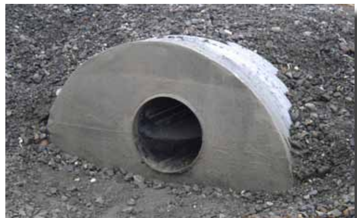
The installation is complete. The culvert is lined with Snap-Tite® pipe and the annular space is filled in with high-pressure grout.
