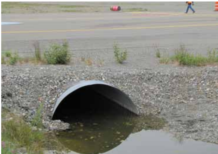
The CMP buckeling under the pressure of the traffic on the taxiway.
