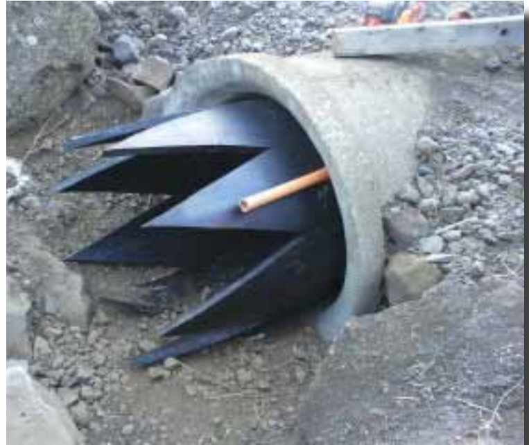
A nose cone coming through the pipe.
