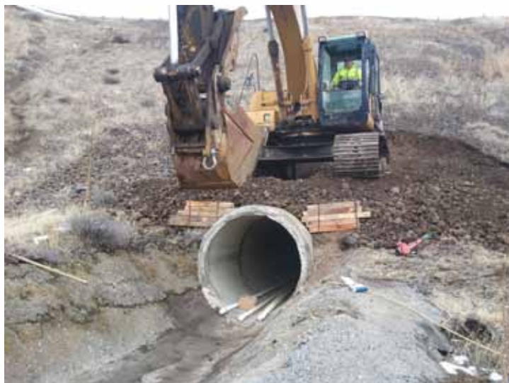
Just prior to the securing of the grout tubes.
