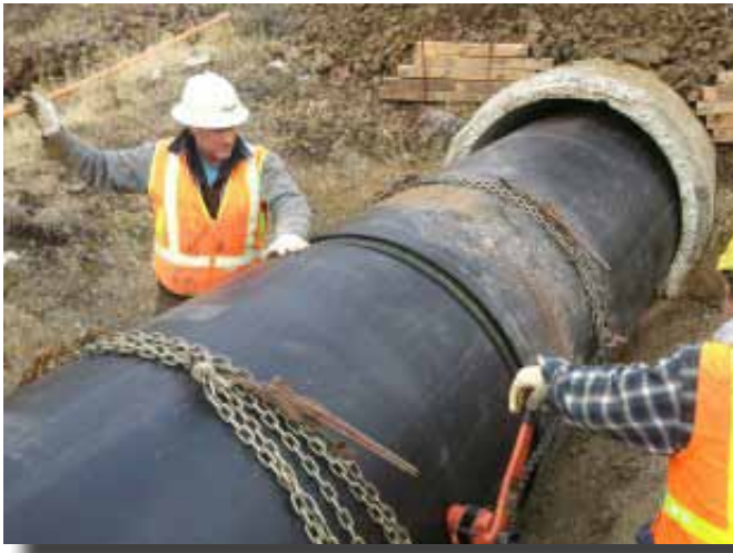
The Snap-Tite pipe during installation.
